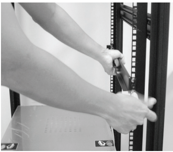
1. Secure the side rails to the rack.
