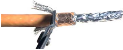
③.paste copper foil on the braided and ground wire and cut off the excess weave and the ground wire
